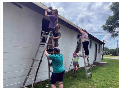
Working together to install new fascia board on a residential home.
